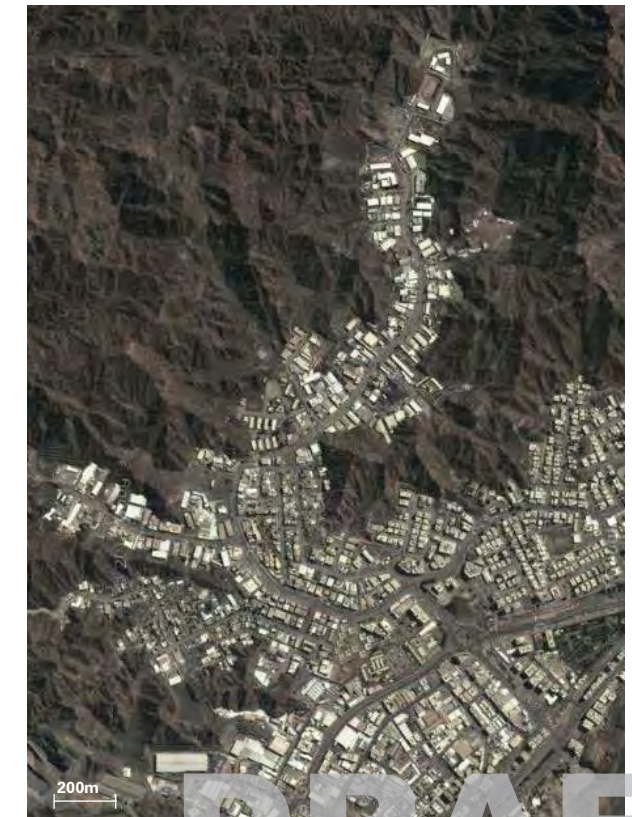
Wadi al Kabir: Built into the Mountains
