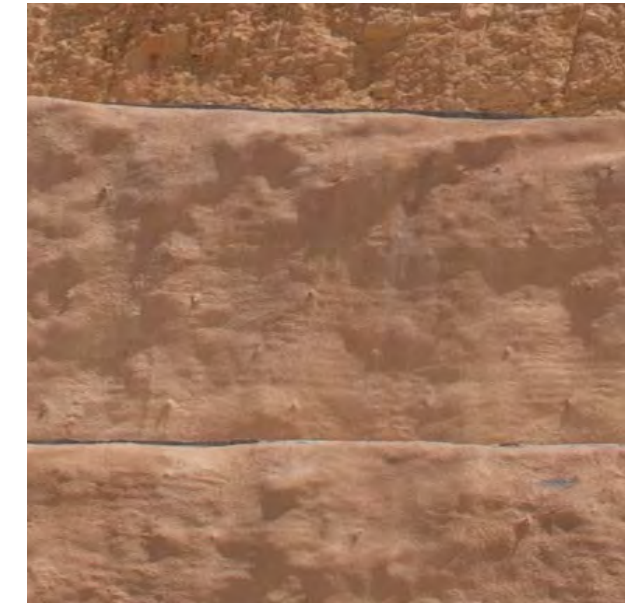
Shotcrete with Weepholes
