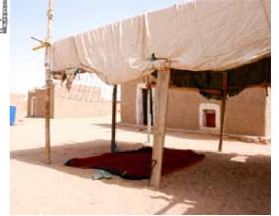
court area, special construction for shade
