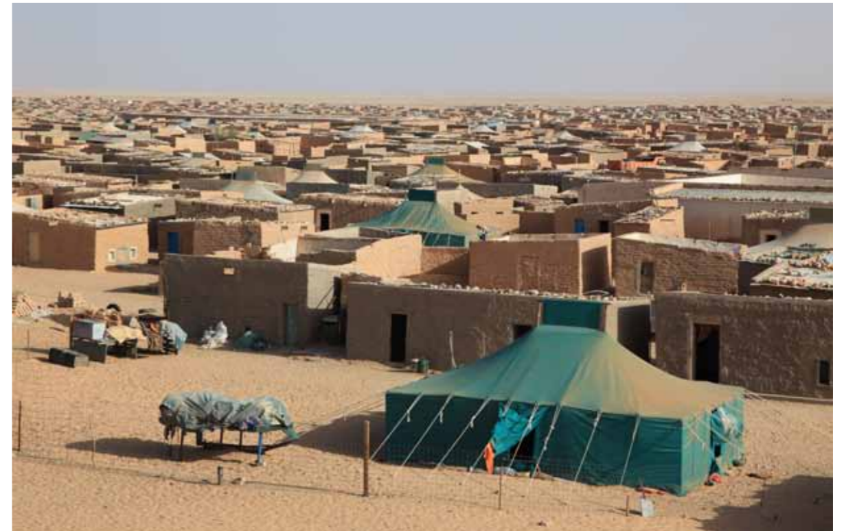
Khaymas integrated in the housing compounds, also being a political statement, Smara 2011 (photo: Manuel Herz)
