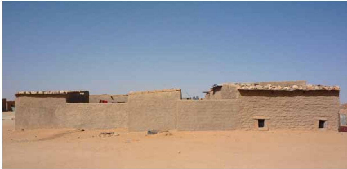
Cement plastered house
