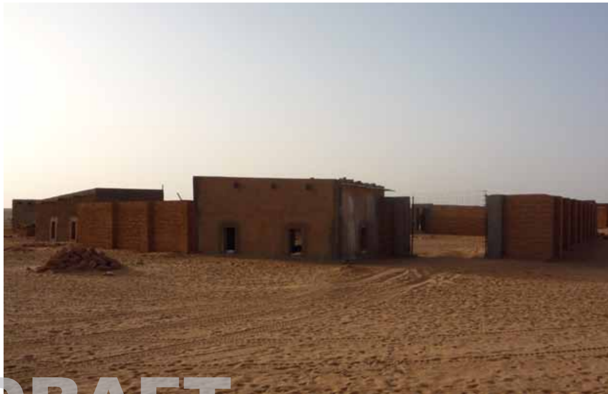
large sized residential compound with a gate
