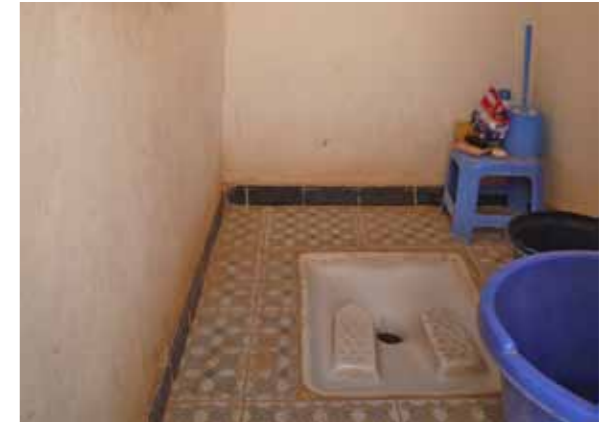
tiled and plasterd toilet
