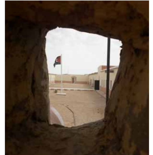
Hole in the wall for water supply
