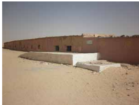
Ramp for Water Supply
