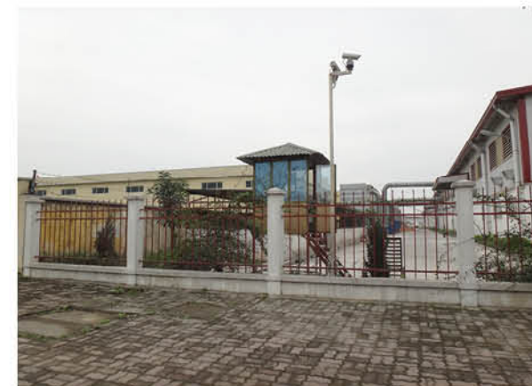
5) factory guard tower and site fences
