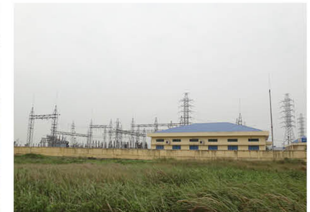
4) power substation, sewage plant
