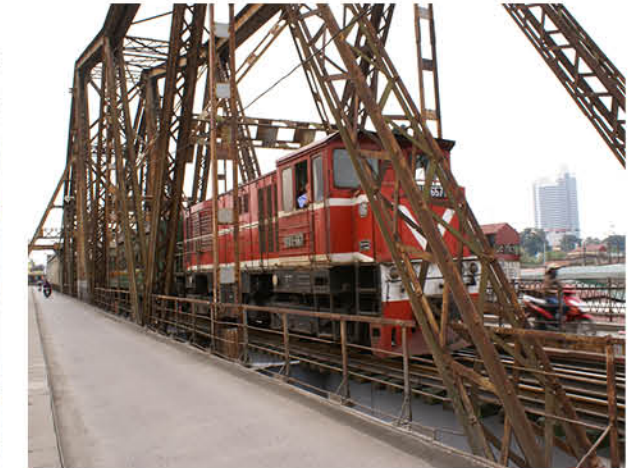
Double-track railway on the Long Bien bridge
