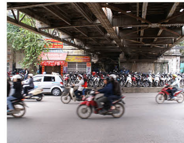
Main road under the Long Bien bridge
