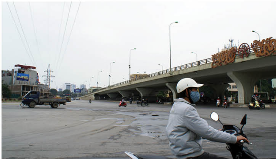
Crossover by national Road in Cau Giay District
