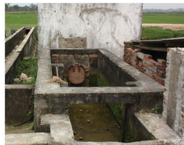
3 Pumping station - Can Co - irrigation and drainage
