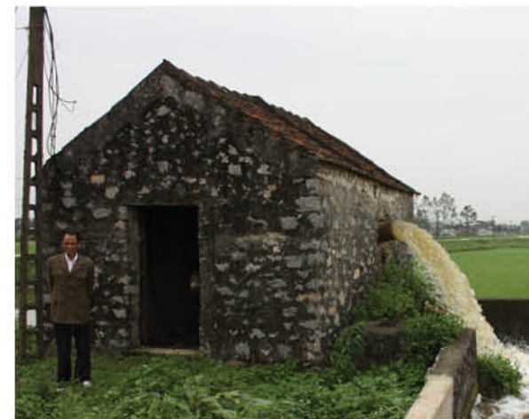
1 Pumping station - Den To - irrigation
