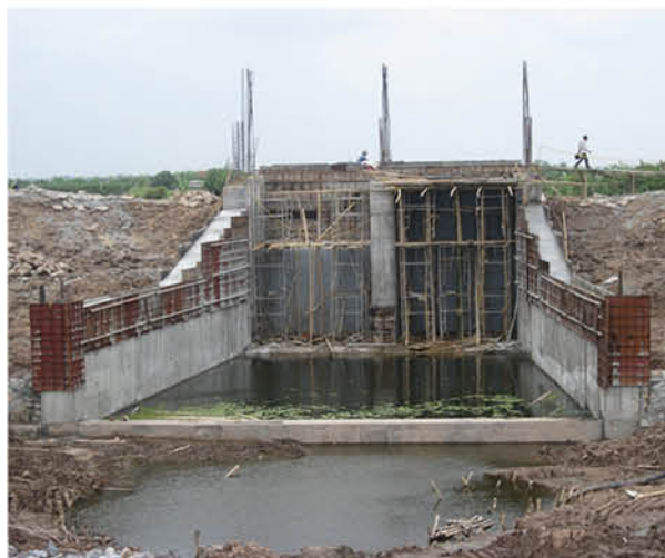
Sluice under construction - Nam Dinh province
