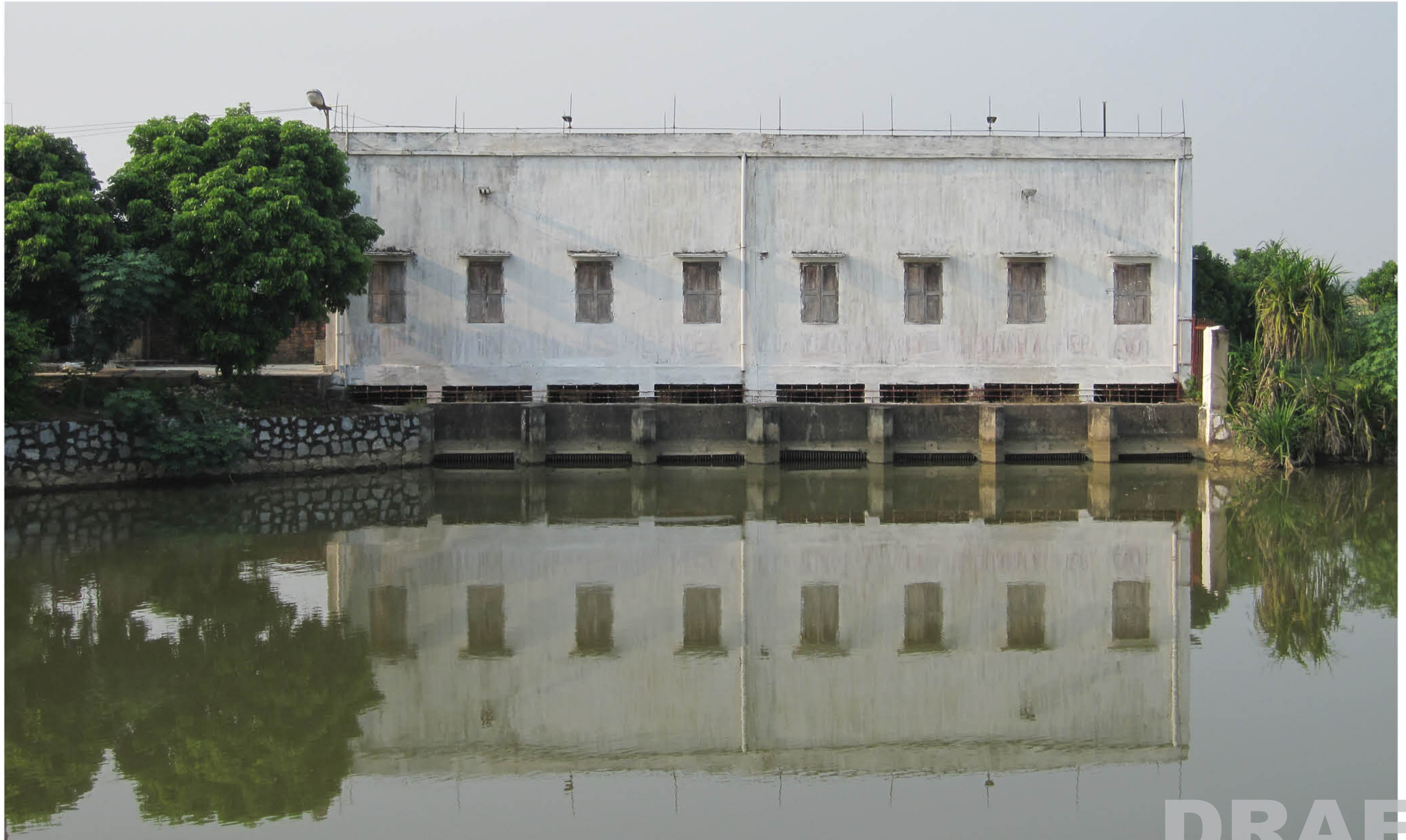
Big pumping station - Nam Dinh Province
