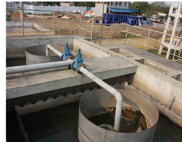
2 Treatment basins with filter
