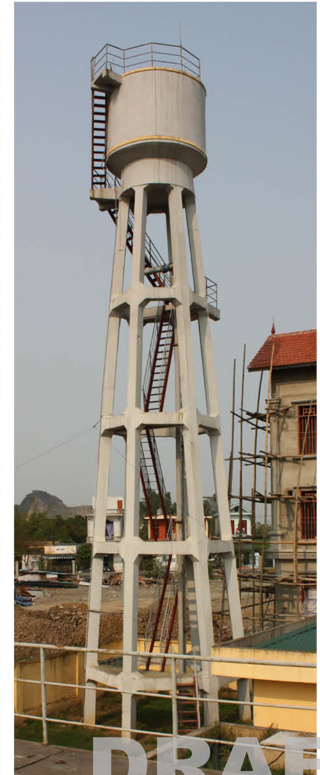
4 Water tower tank
