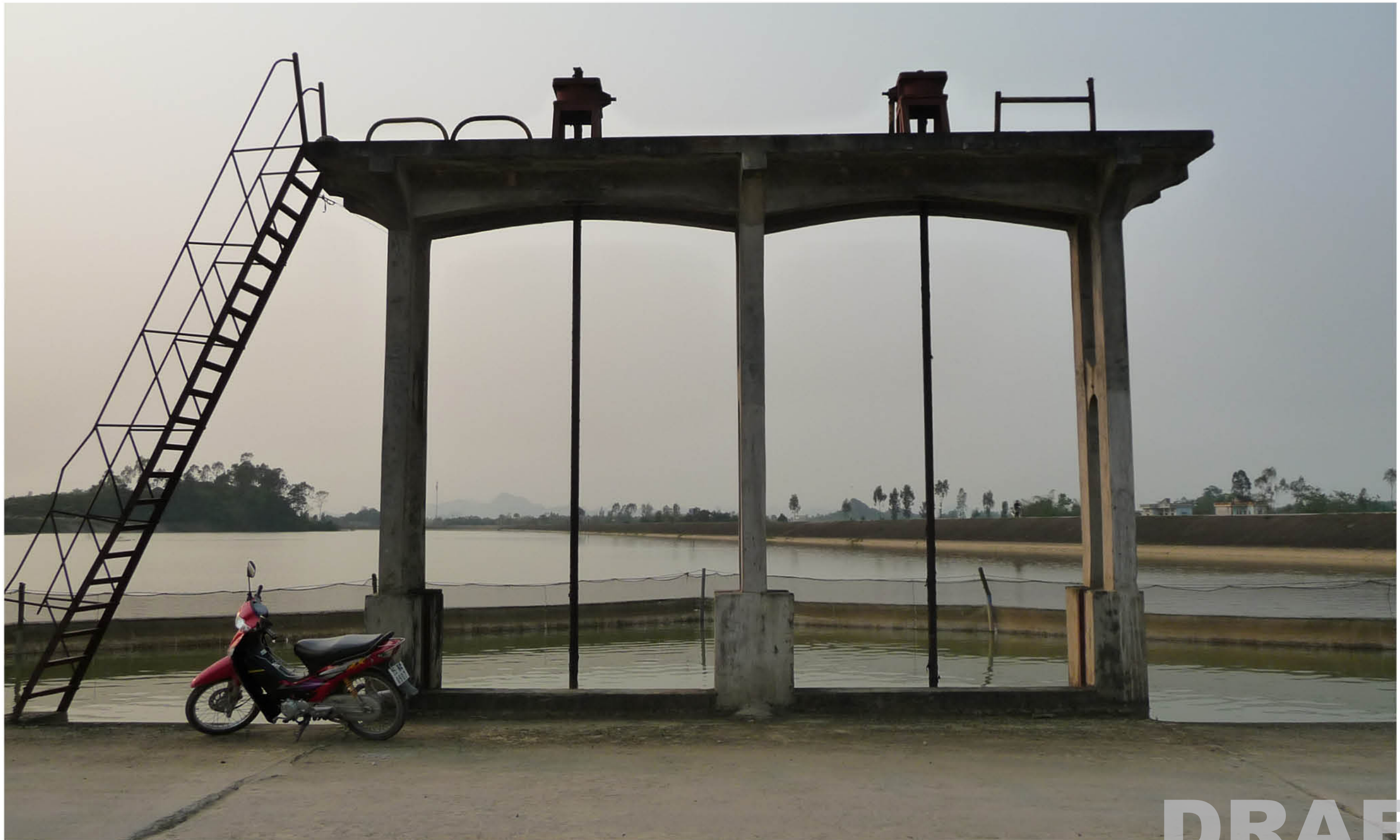
Sluice at the lake Yen Thang - Ninh Binh Province
