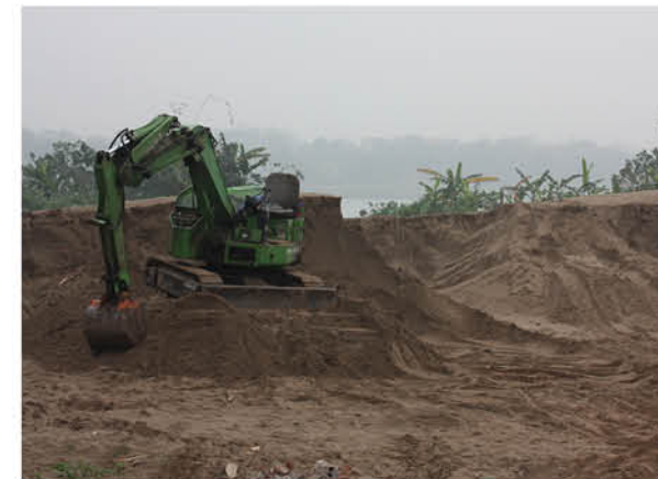
Processing of drilled sand for the market
