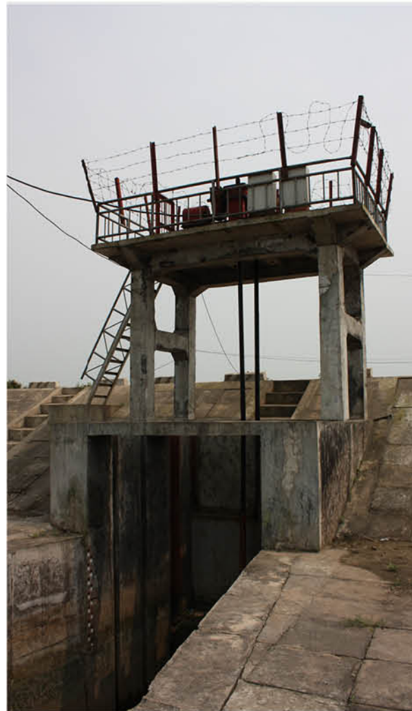
Sluice category I
