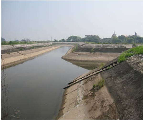
Main Canal KC
