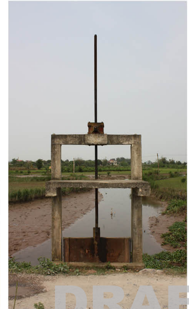
Sluice category II
