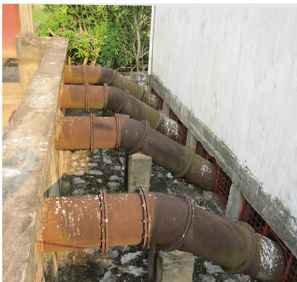
Old pumping station - Nam Dinh province
