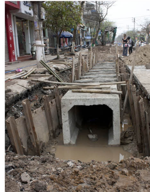
Drainage under construction - Nam Dinh City
