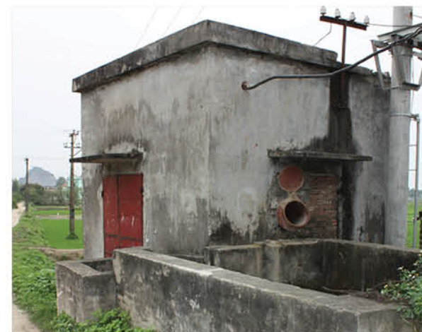
2 Pumping station - Dong Dam - irrigation and drainage
