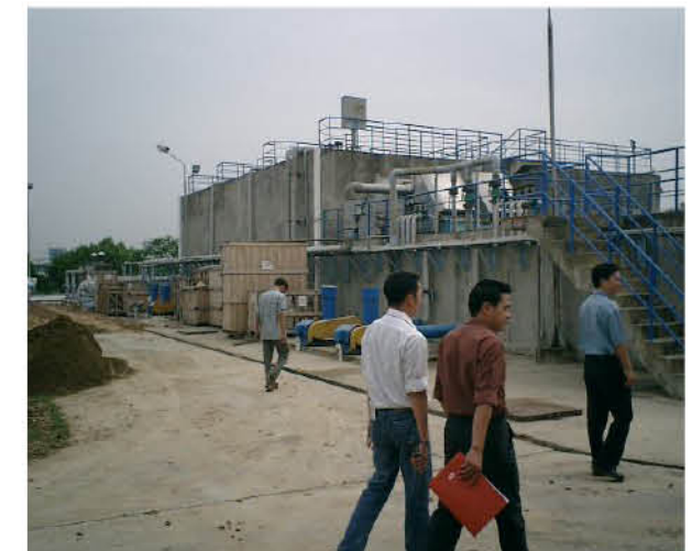
Treatment plant of an industrial park
